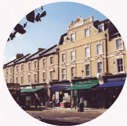
SHOP FRONT IMPROVEMENTS A successful heritage economic regeneration scheme in Forest Gate, east London
