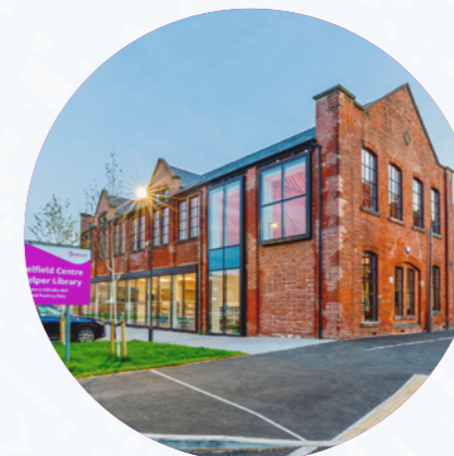
ADA BELFIELD CENTRE, BELPER Former Thornton's factory in Derbyshire, re-purposed as a residential care home and public library
