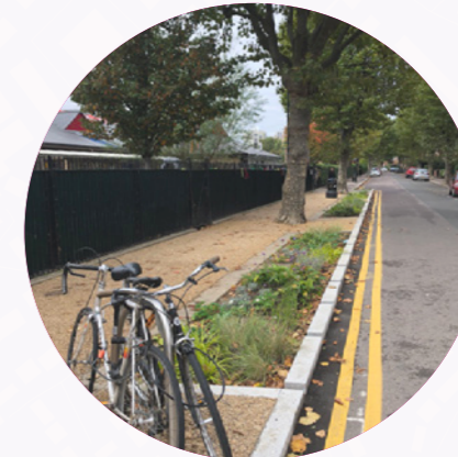
PAVEMENT WIDENING Resurfacing, planting and bike storage to improve walking and cycling facilities in north London.
