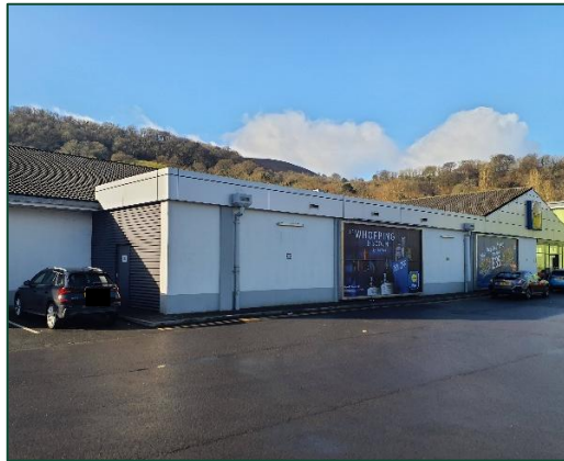
IMAGE 4 – DEVELOPED LAND; SEALED SURFACE (BUILDING)
