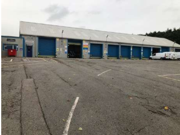
Photo 1: A view north showing the existing bus depot, taken from the centre of the proposed store.
