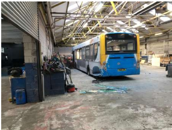
Photo 3: Photograph displaying the rear of the bus depot, where a body shop is located, in the northernmost section of the site, view looking west (taken from the centre of the northern section of the site).
