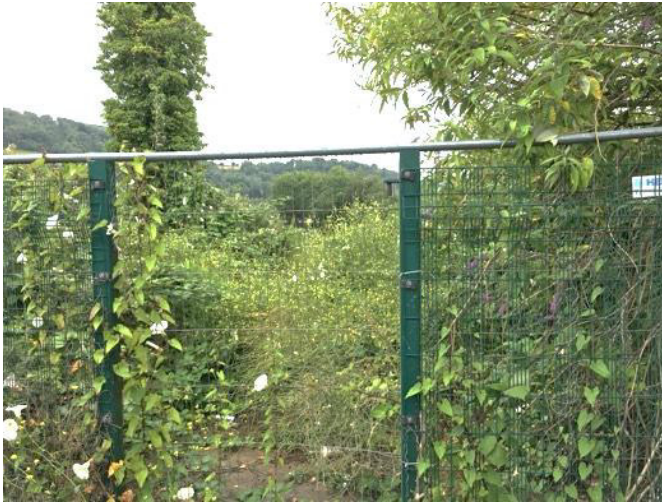
Photo 7: Evidence of overgrown vegetation in area on west side of public footpath
