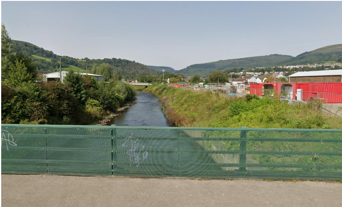
Streetview Image at the road bridge on the B4591 (NGR 324437, 189789) facing upstream (adjacent to site boundary). Image extracted on 24/10/2024.
