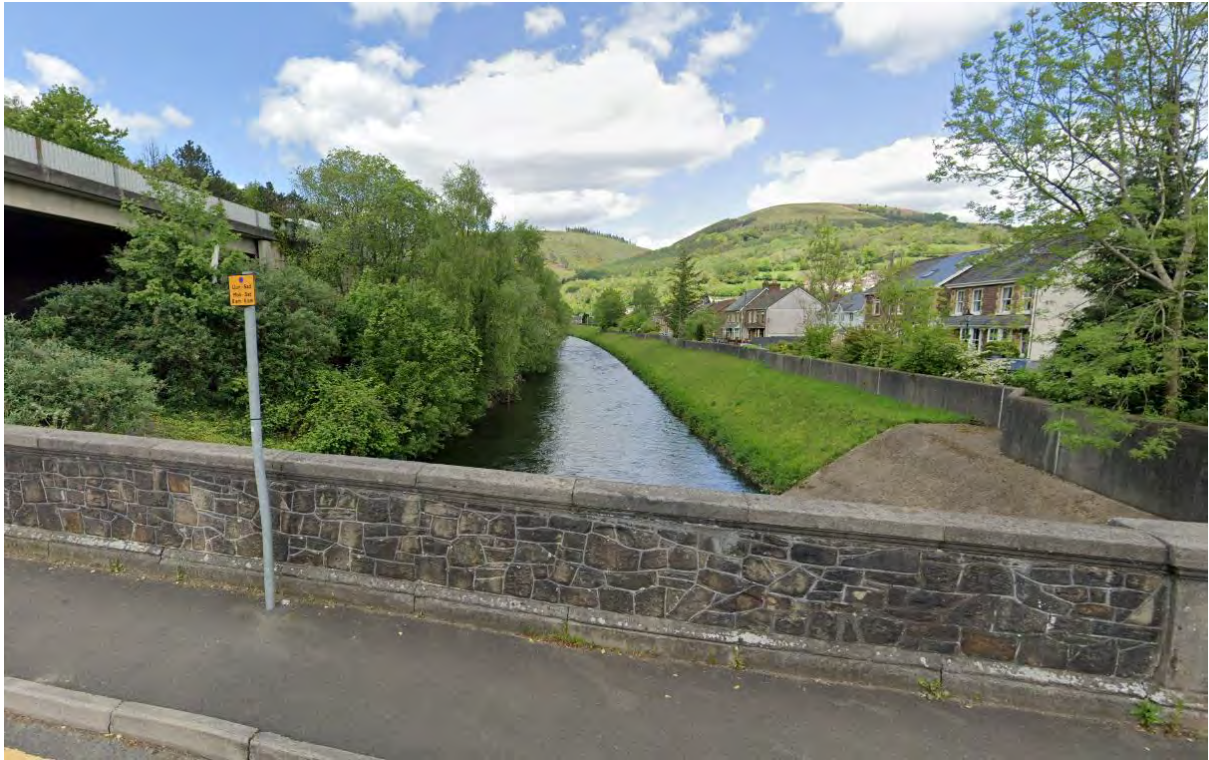
Streetview Image at the bridge on Dan y Graig Road (NGR 323621,190544) facing upstream. Image extracted on 24/10/2024
