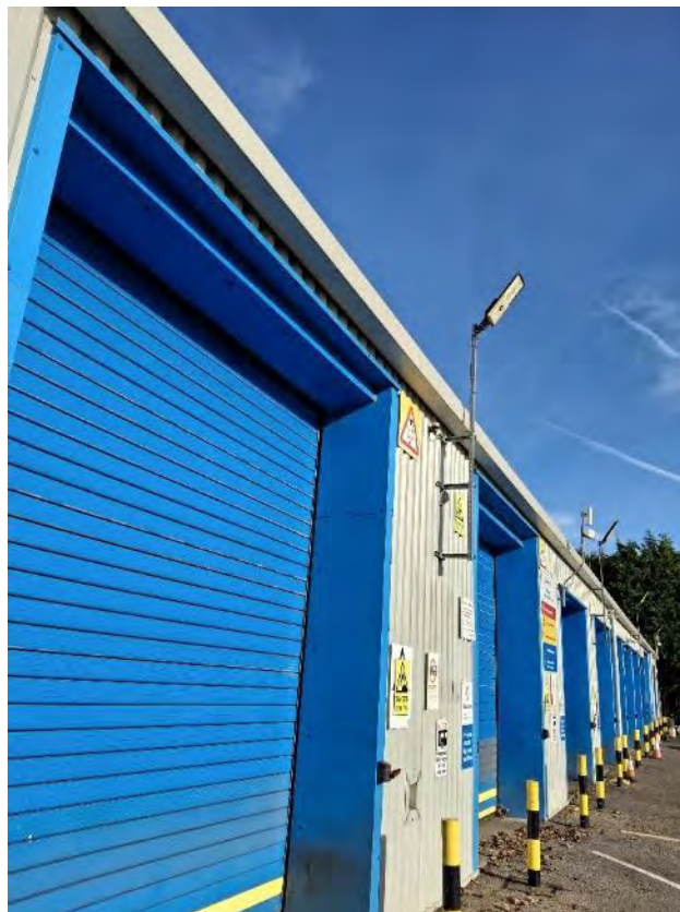
Photograph 12 – Building A: South aspect of warehouse. Shutter doors located to the rear to allow buses to enter and be repaired
