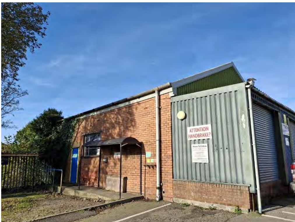
Photograph 14 – Building B: South aspect of smaller storage building. Single storey with a pitched roof and brick walls
