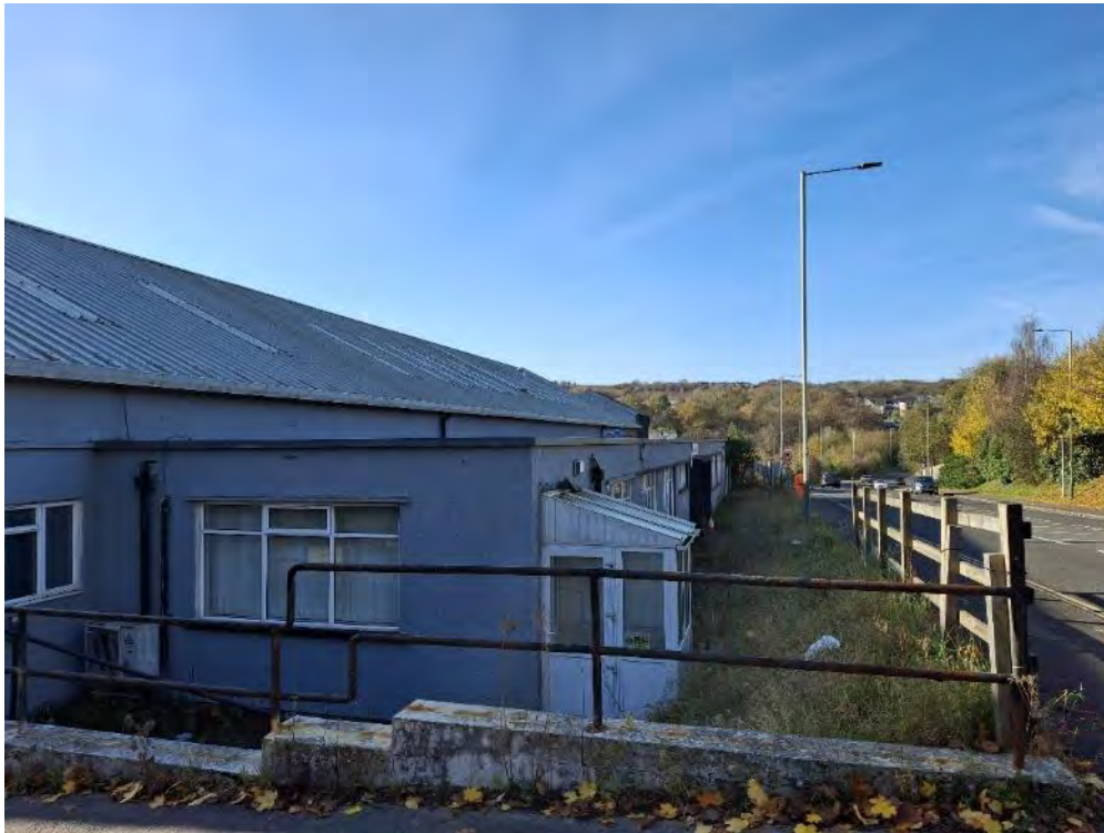
Photograph 11 – Building A: North aspect (front) of warehouse depot beside B4254 road
